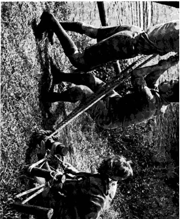
The ends of hand ropes to the first stakes on each side of river with two turns and two half hitches. Go over all the ropes, tightening them as much as possible. Your bridge is done, ready for crossing.
